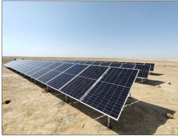
Fig 1: Monocrystalline P.V panel with 0.8 meters above the ground with 580 watt power.
